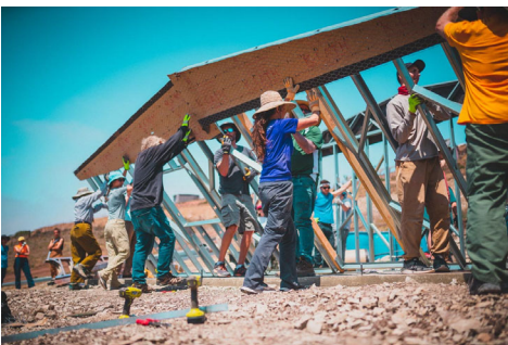
Project Mexico volunteers screw together metal frames to form the walls for a new house.
