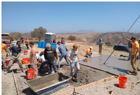
Halfway through the first day of work, you can see the concrete foundation taking shape.
